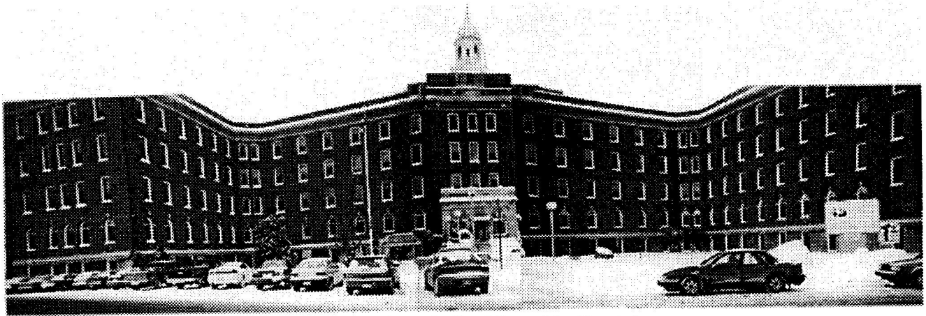
Figure 1. East View of the Hospital
